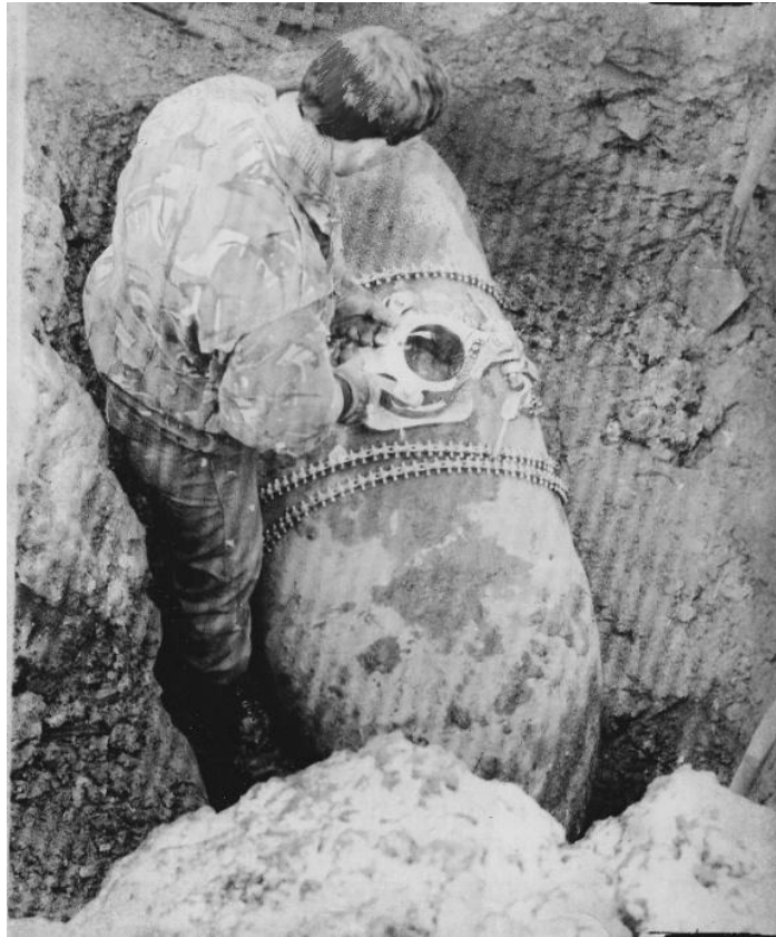
Sheffield 1985, Trepanner being fitted to the UXB.
