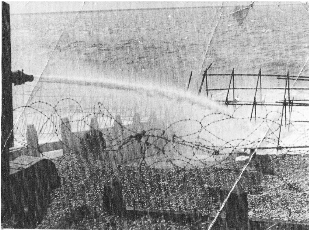
High Pressure Water Jetting use to uncover Beach Mines laid as anti-invasion measures between 1940 and 1942. Brighton Beach.
